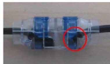
Wires terminated correctly
